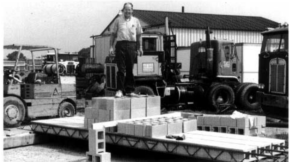
Testing for construction loads on an ungrouted assembly
